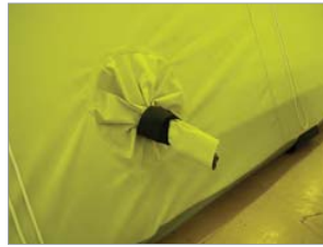
Opening for heating
